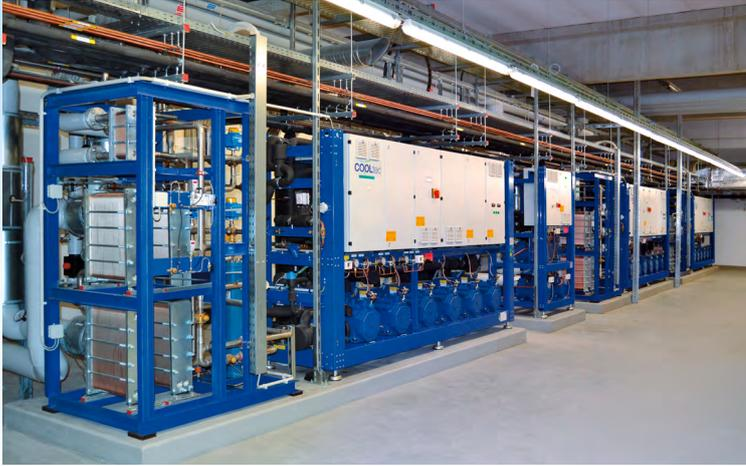
Latest generation of CO<sub>2</sub> transcritical systems, CO<sub>2</sub>OLtecEvo® provides energy efficient and environmentally sustainable refrigeration, through our patented modulating ejector technology and a CO<sub>2</sub> pump.
